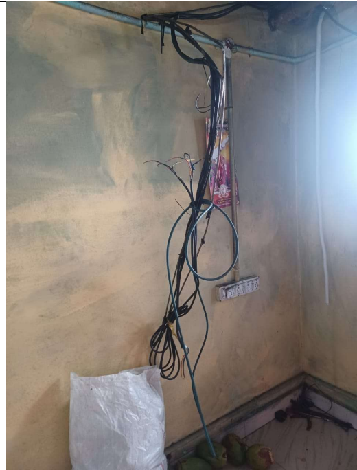
OCEMS (under repair) connected to the stack
